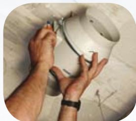
Place the impeller and motor assembly
